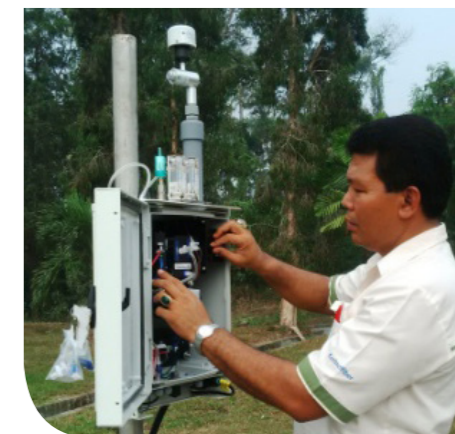
Fire Prevention Manager, Saial Arimi servicing Dust Sentry
