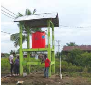
RER provided a 75-meter deep well and 1,000-liter storage tank to serve 50 families in Mayangsari Village to improve the wellbeing of the residents of Pulau Padang by providing the community with clean water and sanitation facilities.
