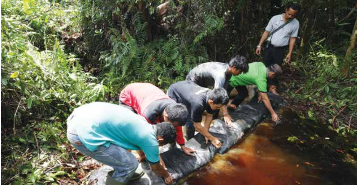
RER has built 25 dams to close nine old drainage canals measuring more than 29km in length in the concessions
