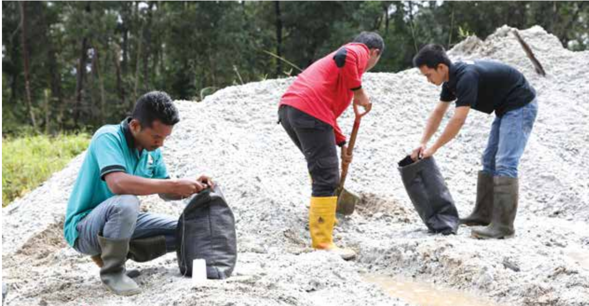
RER teams filling sandbags to be used for blocking canals
